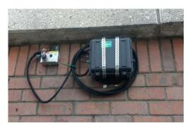
Photo 7: Typical Vibrograph installation
