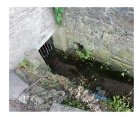
Photo 1.2 & 1.3: Grated Drainage Openings Along the Eastern Boundary
